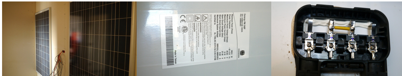
Above photos are of the two PV panels I use as heaters since November 2019 and they work great as expected. You can see the yellow wire soldered in the PV panel connection box to disable the middle 20 cells of the panels leaving the ideal 40 cells in series. Max PV panel temperature here is 50C but the most I see was about +55C so very reasonable.
